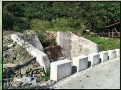
鄉公所施作沉砂池(4M*3.5M)
